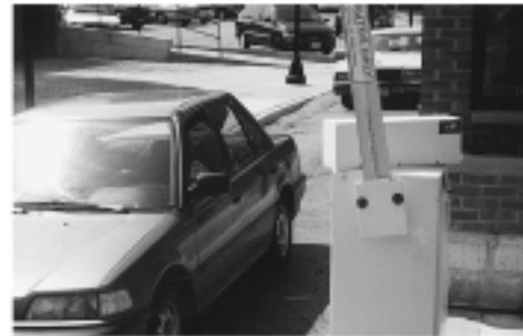
FIGURE 69: A PHOTOELECTRIC SENSOR PREVENTS COMMUTERS FROM FOLLOWING YOU THROUGH THE TOLLBOOTH FOR FREE
